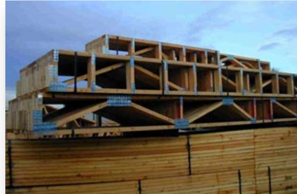
Parallel chord trusses stacked and awaiting delivery
